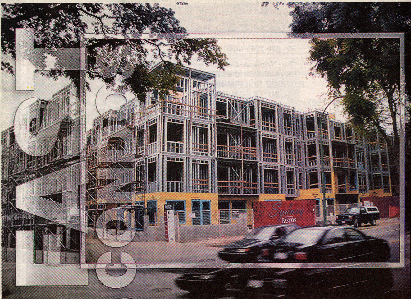
FAST CONDOS: Power MBS Structures Inc. of Langley has developed a super fast pre-fab and engineered light steel and concrete system for building homes and low-rise residential buildings. The MBS system involves 12-gauge to 20-gauge galvanized steel and an open web steel joist floor system. Shown is a Bastion Development project in Vancouver completed with the MBS system. Photos: Power MBS
